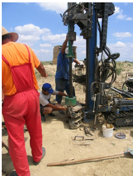
Geotechnical investigations at Saligny
