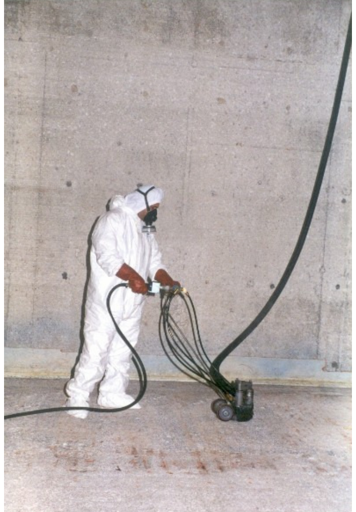
Spent fuel pool decontamination
