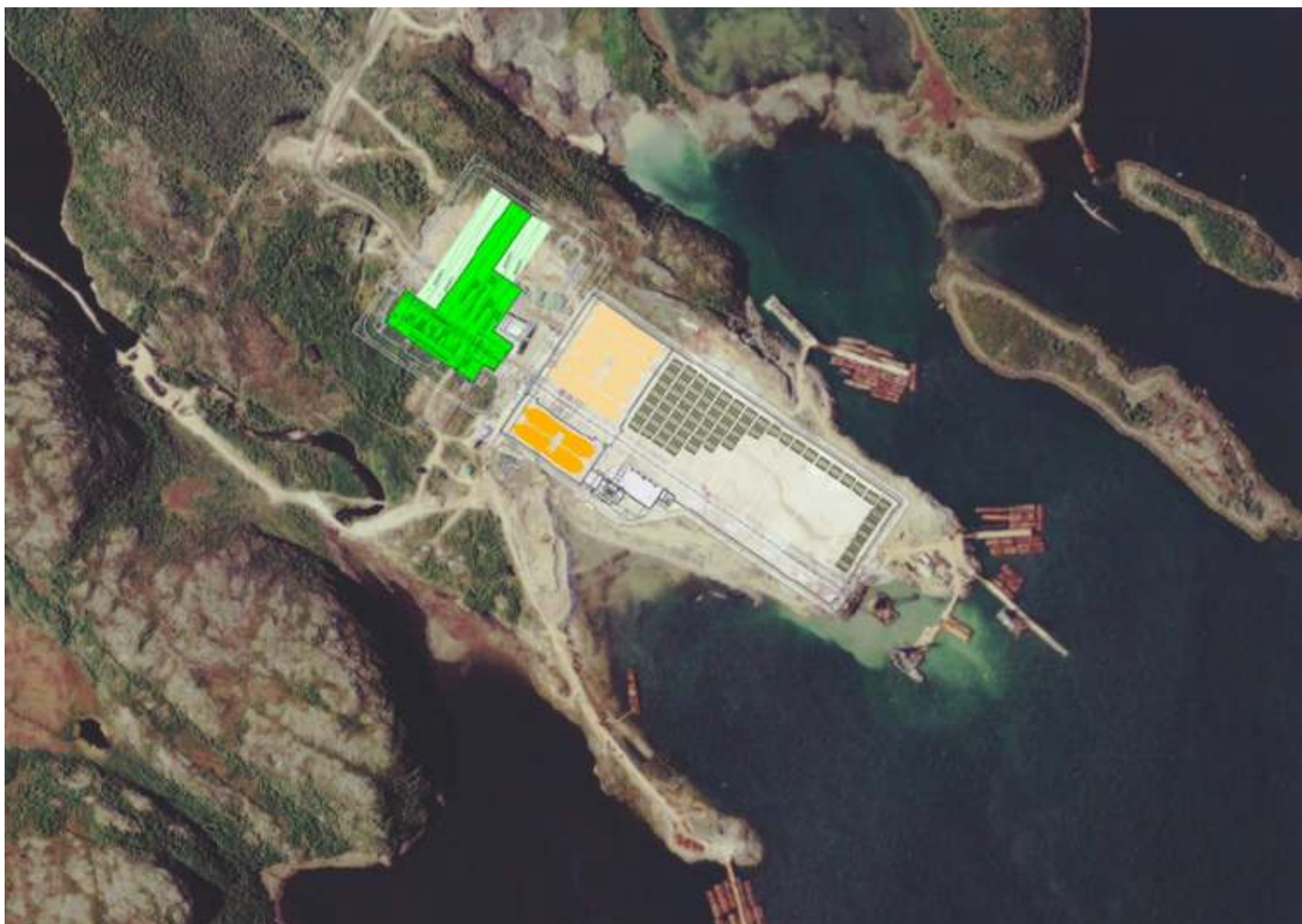
Saida Bay Facility from above: green — the future centre for radioactive waste treatment and storage; yellow – storage for contaminated service ships (under construction); black – storage for submarine reactor units (completed)
