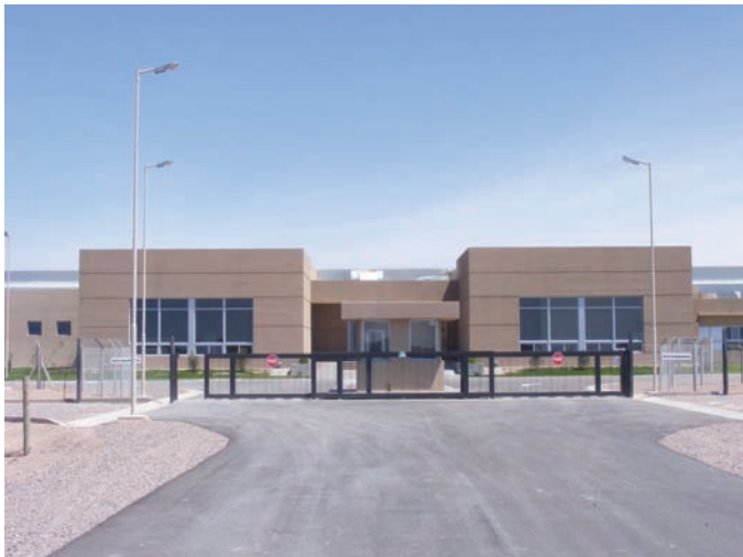
The new multi-purpose insect rearing facility in Mendoza, Argentina.
