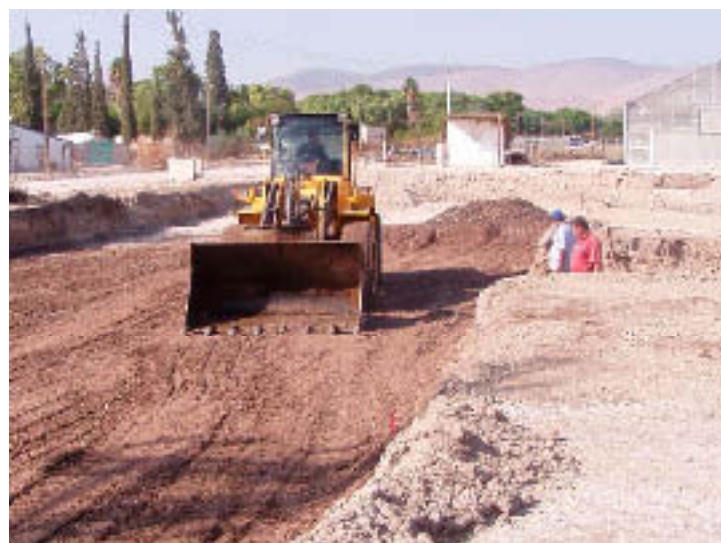
Fig. 10: A caterpillar starting first operations aiming at constructing the first private medfly rearing facility ever in the Middle East
