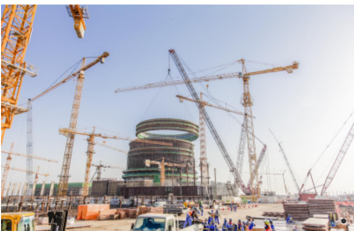
Construction work at the Barakah NPP, August 2014 (Photo Credit: Emirates Nuclear Energy Corporation/IAEA)
