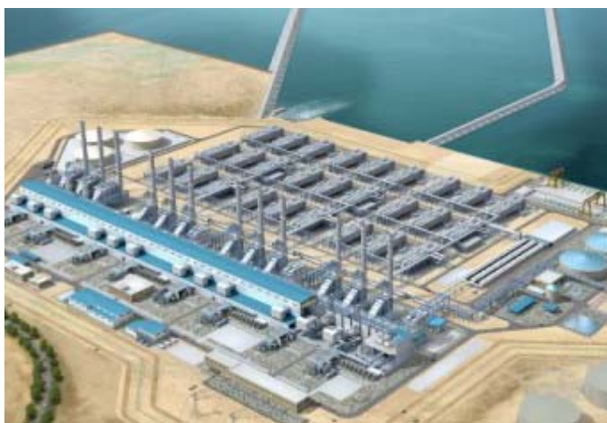
Jubail II thermal desalination plant in Saudi Arabia
