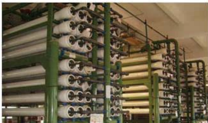
SWRO desalination plant in Hongyanhe nuclear power plant
