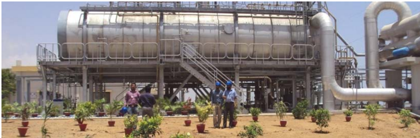
Karachi nuclear desalination demonstration plant
