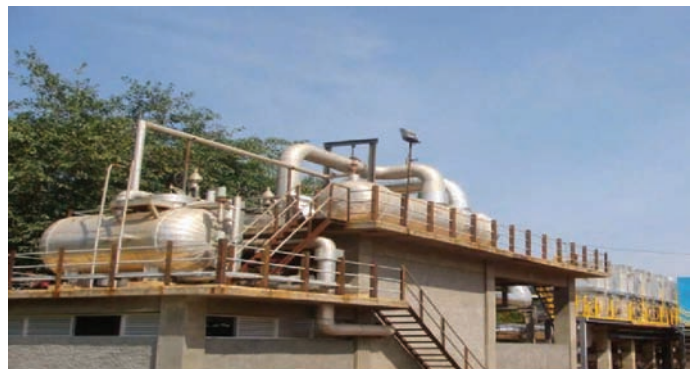
Kalpakkam Nuclear Desalination Demonstration Plant
