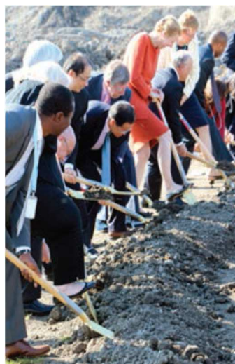
Participants join DG in the groundbreaking
