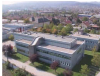
AGES facility in Mödling
