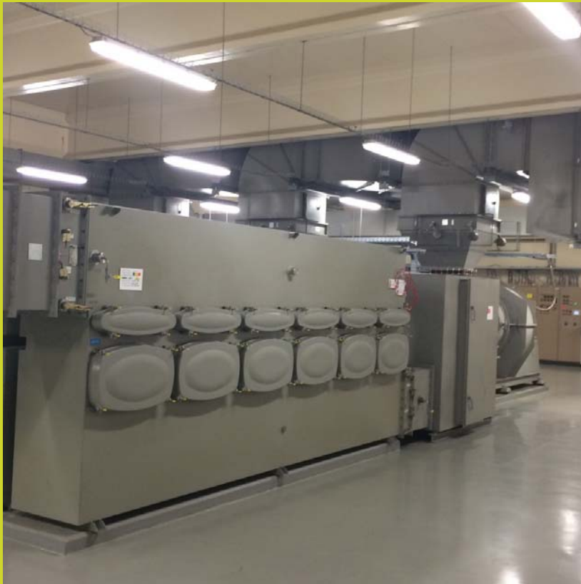
Hepa filter bank and extraction fan
