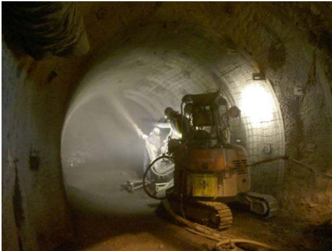
Shotcreting test at Horonobe URL
