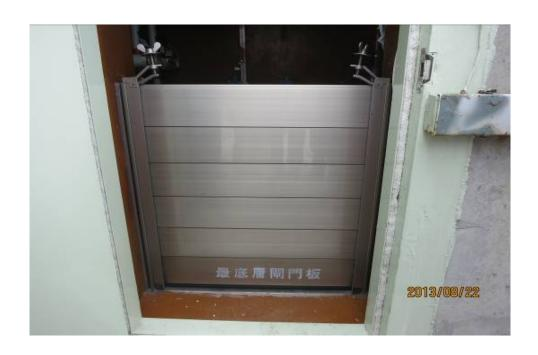
Flash boards on border gates of key building – Tianwan NPP, China
