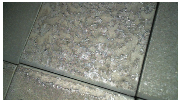
Figure 9: Example of the degradation of the boron film on molybdenum tiles on the outer divertor. Note the middle tile has degraded but the tile to the left and right are as installed.
