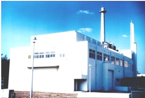
Actinide research facility Oarai branch, Tohoku Uni.
