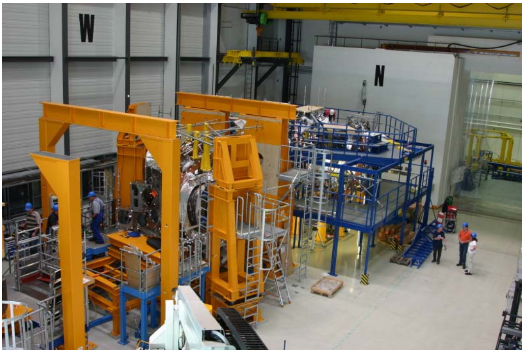
FIG. 4. First two assembly stands for the pre-assembly of the magnet system, the installation of the support elements and part of the Helium pipes and the bus bar system.
